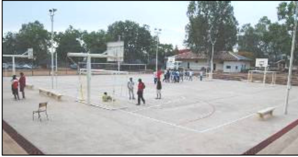
Western view of basketball courts and bleachers to be covered by the roof.
